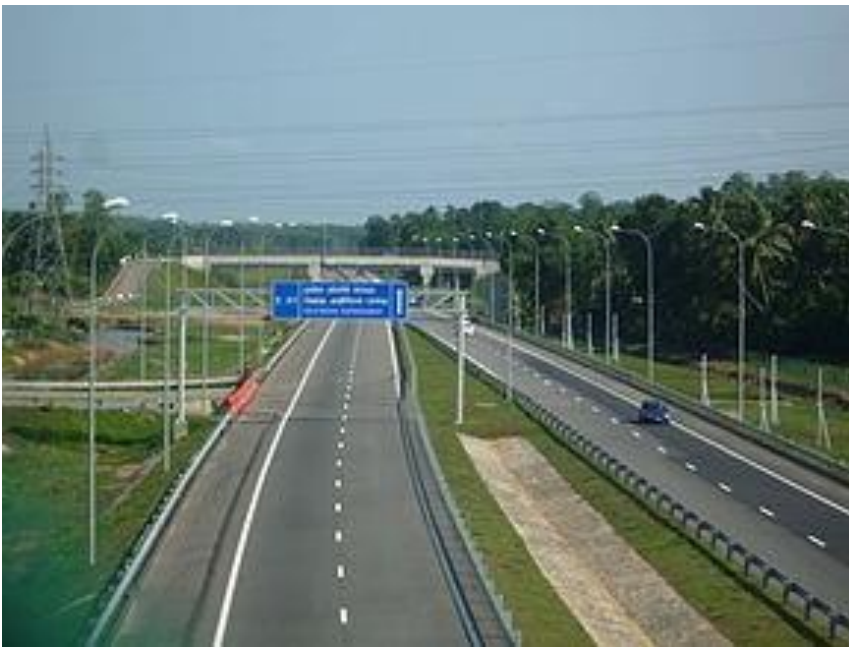
Sri Lanka's Southern Expressway, its first major highway
